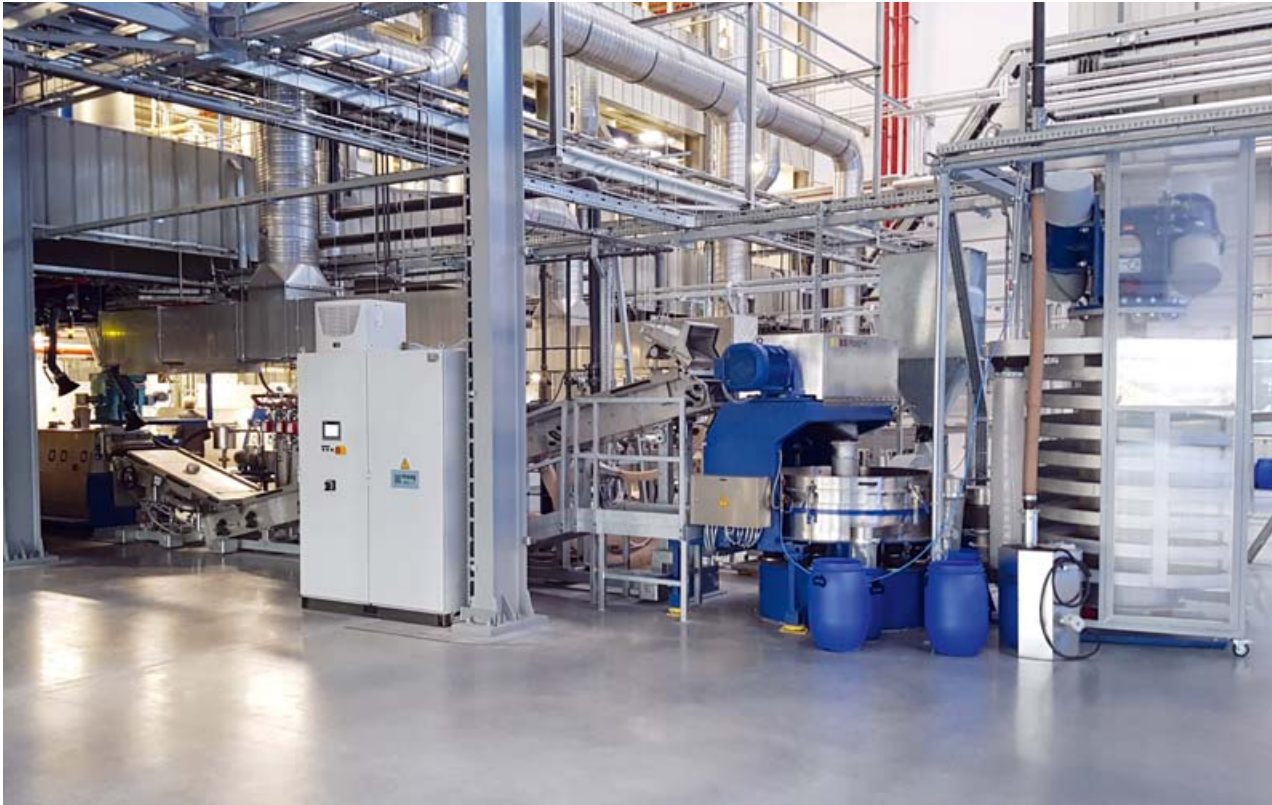
JSG 400 with classifier and spiral conveyor
